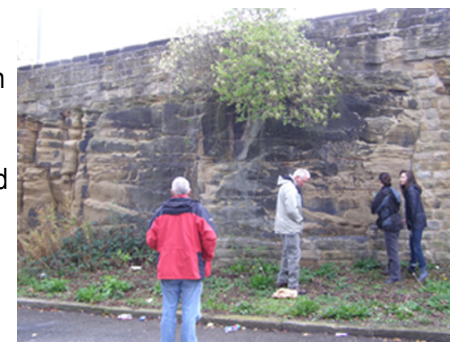
Surveying in Ackworth Moor Top quarry
