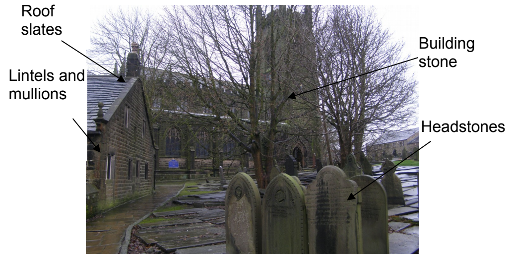
Heptonstall churchyard to show the use of local sandstones
